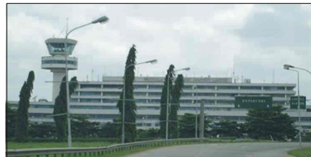
Murtala Mohammed International Airport Road, Lagos
