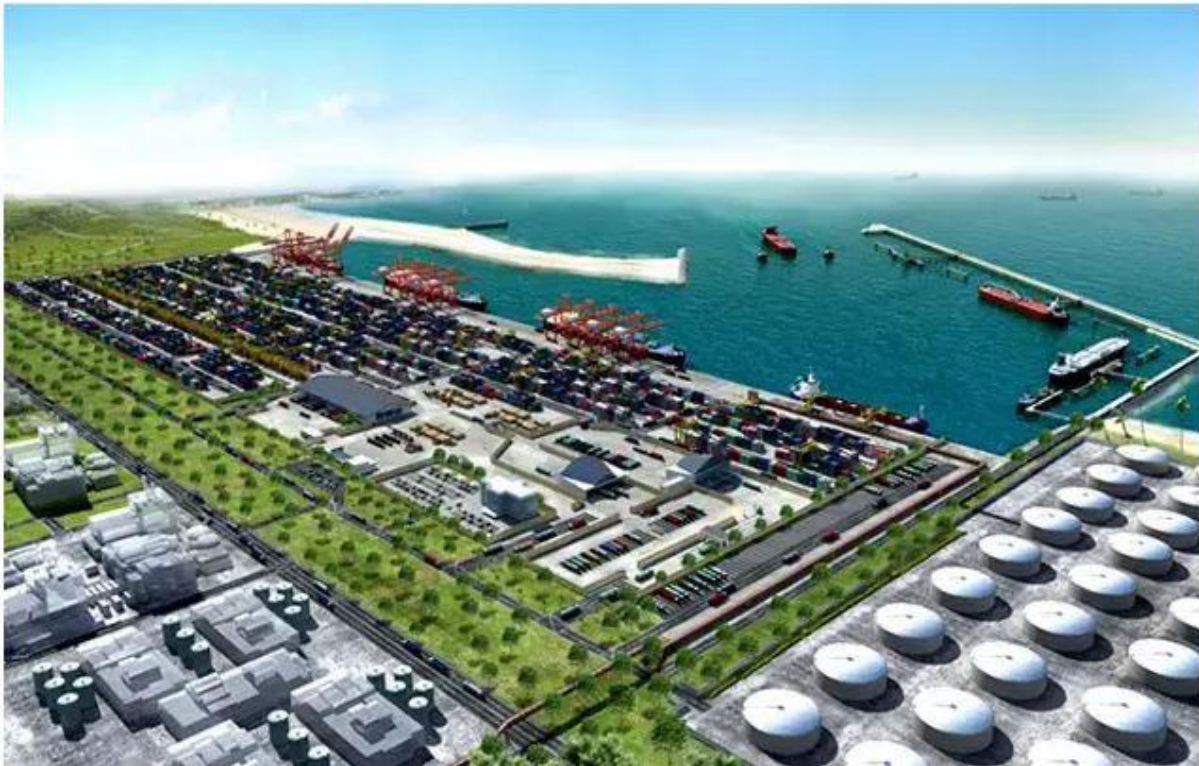
Badagry Deep Sea Port - Photo Source Construction Review online
