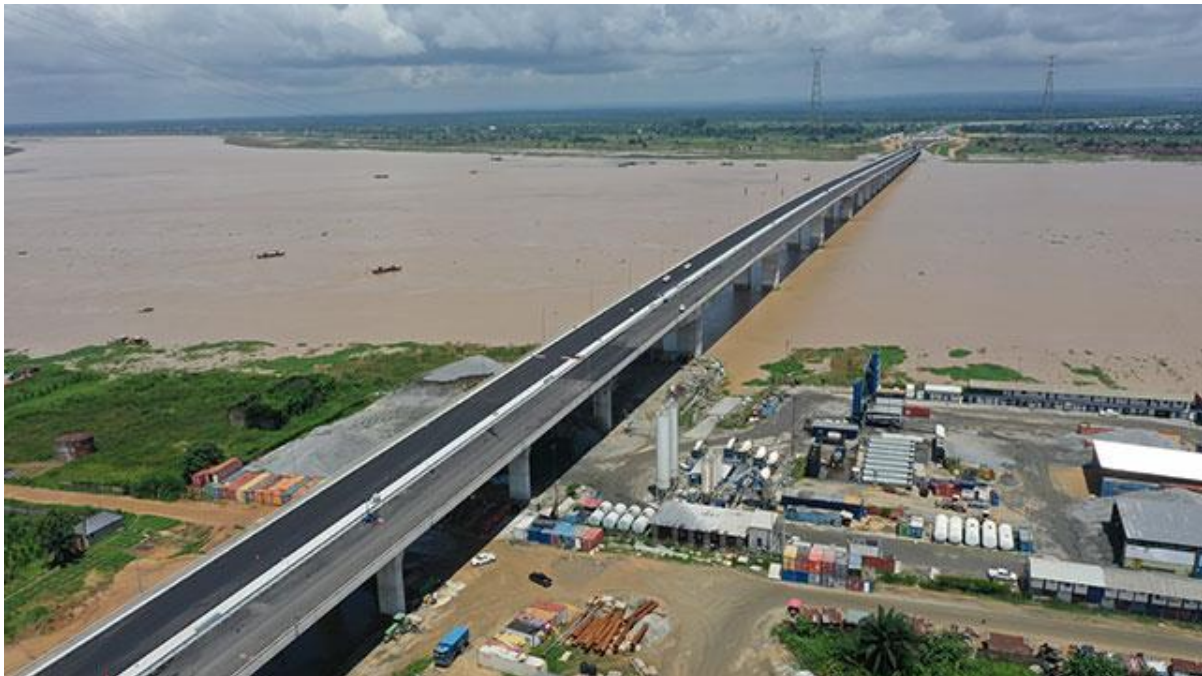
Second Niger Bridge Photo source - Julius Berger
